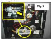
Water heater drain plug location
