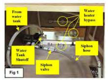
Water valves and water heater bypass
