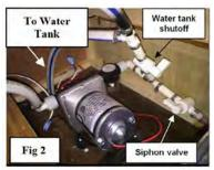
pump will run and pressurize the water lines, and water should flow from the fixture.
