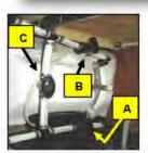
Factory installed 3-valve water heater bypass
