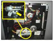
Water Heater Drain Plug Location
