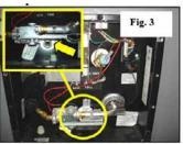
Water heater drain plug location
