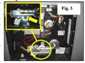
Water heater drain plug location
