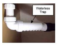
ing to open the drain. Passing a cleanout tool through the waterless valve may cause damage to the internal seal that may potentially allow sewer gases to escape into the RV interior. The waterless trap can be unscrewed from the water lines. A label has been placed near the location of the waste valve that reads as follows:
