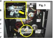
Water heater drain plug location
