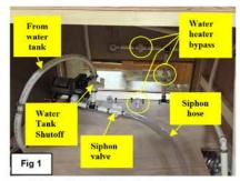
Water valves and water heater bypass
