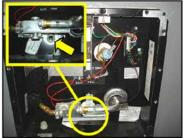
Water Heater Drain Plug Location
