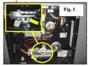
Water heater drain plug location
