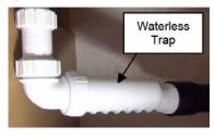
gases to escape into the RV interior. The waterless trap can be unscrewed from the water lines. A label has been placed near the location of the waste valve that reads as follows:
