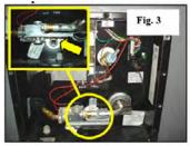
Water heater drain plug location
