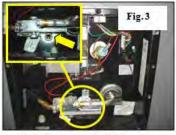
Water heater drain plug location
