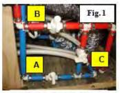
Factory Installed 3-Valve Water Heater
