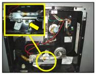
Water heater drain plug location
