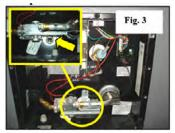
Water heater drain plug location
