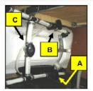
Factory installed 3-valve water heater bypass
