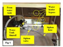
Water valves and water heater bypass
