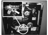
Water heater drain plug location
