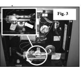
Water heater drain plug location
