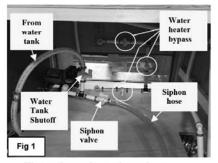
Water valves and water heater bypass
