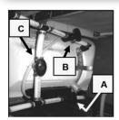
Factory installed 3-valve water heater bypass
