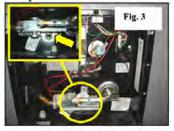
Water heater drain plug location
