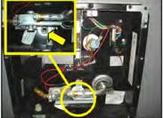
Water Heater Drain Plug Location
