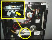
Water Heater Drain Plug Location
