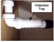
damage to the internal seal that may potentially allow sewer gases to escape into the RV interior. The waterless trap can be unscrewed from the water lines.
