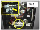
Water heater drain plug location
