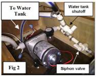
the fixtures. When a fixture is opened, the pump will run and pressurize the water lines, and water should flow from the fixture.
