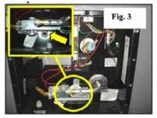
Water heater drain plug location
