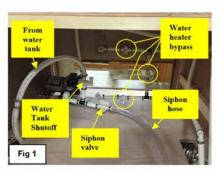
Water valves and water heater bypass
