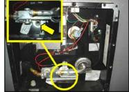
Water Heater Drain Plug Location
